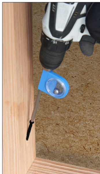
Typical WSTS45-EXT stud to bottom plate installation
