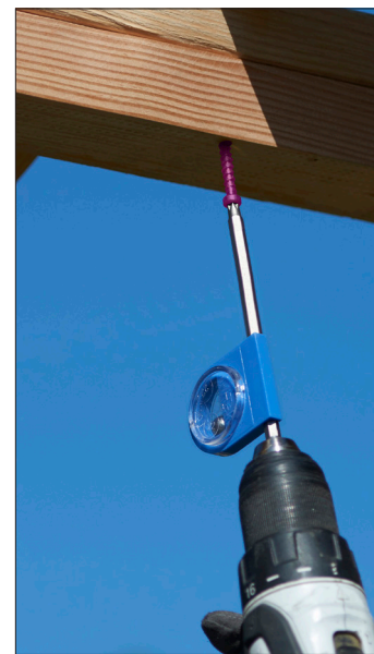
Typical WSTS6-EXT truss to top plate installation
